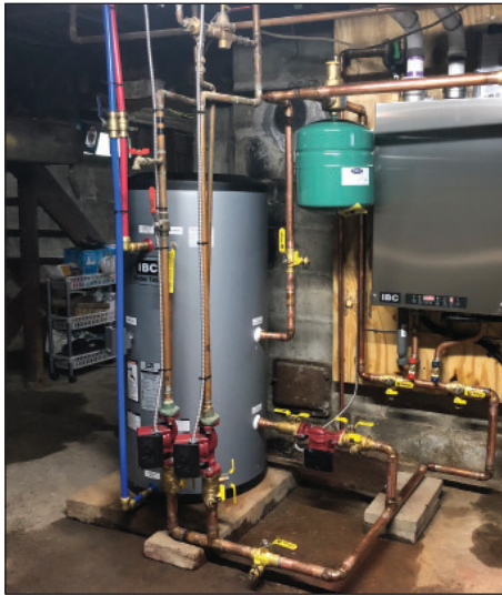
Energy Services converted an electric hot water tank and an oil furnace to an energy-efficient natural gas boiler system for a weatherization participant.
