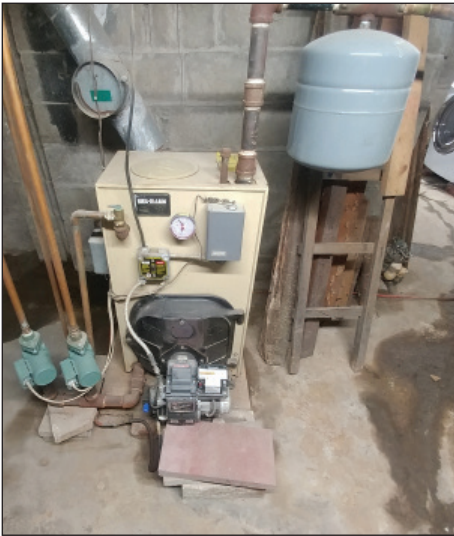
Energy Services converted an electric hot water tank and an oil furnace to an energy-efficient natural gas boiler system for a weatherization participant.
